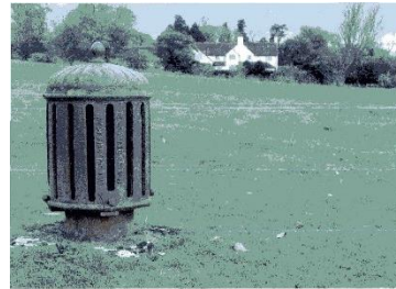
Ventilator for water reservoir. Photo: Brian Lewis
